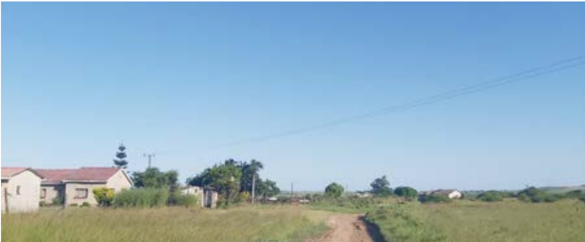
Figure 1. 10: Lattice Structure No 21 , Showing the current land use on site, facing eastern direction towards the residential house in close proximity of structure 21.
